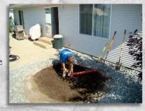
Position belting to separate the cement blocks from the rubber liner below.
