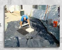
Trim away the excess liner and felt materials. Spread the rocks out to completely cover the liner.
