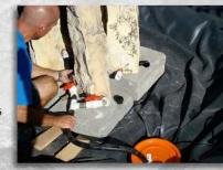
Dig the hole 12 to 18 inches deep so ample water will circulate to the pump.
